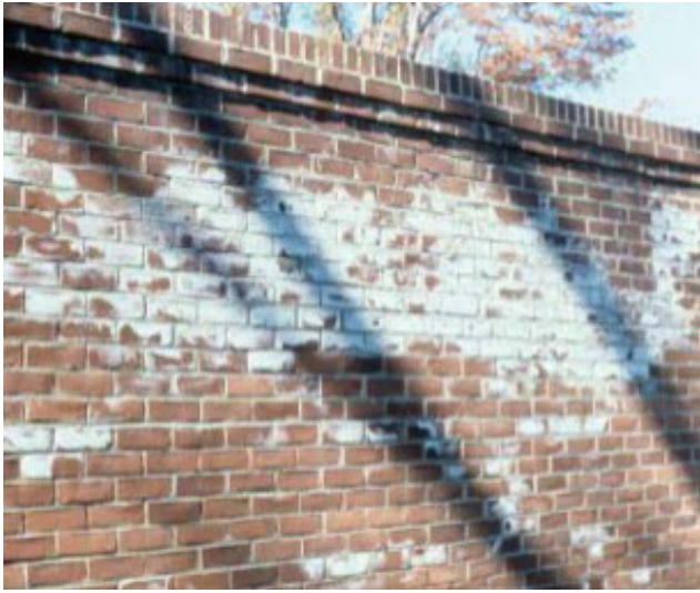
Photo 1 Efflorescence
