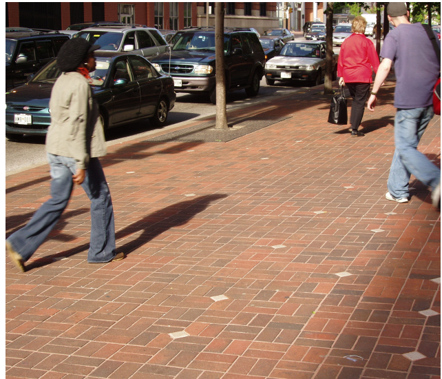
Photo 4 Clay Paver Sidewalk in Basket Weave Pattern
