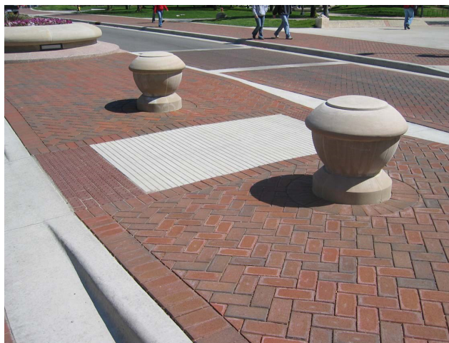
Photo 5 At-Grade Street Crossing with ADA-Compliant Surface Texture Changes
